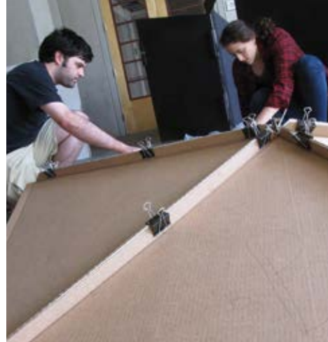
Physics and astronomy graduate students Kevin Fogarty (left) and Alexandra Greenbaum assemble the dome of the planetarium, made of cardboard triangles and attached with binder clips, for easy assembly.
